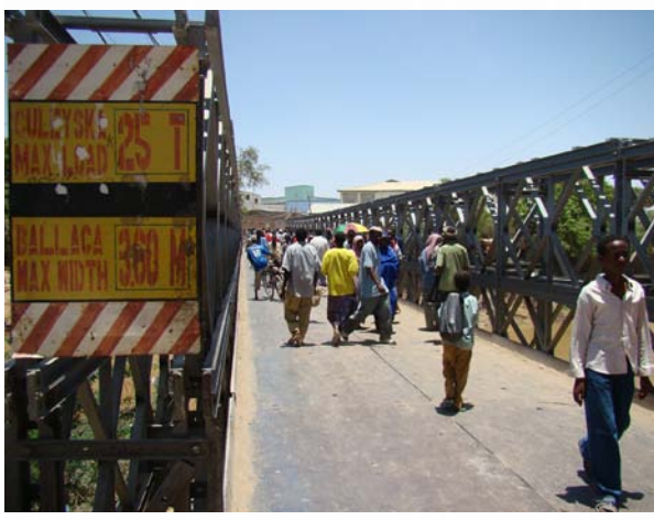
Buundo Weyne bridge
